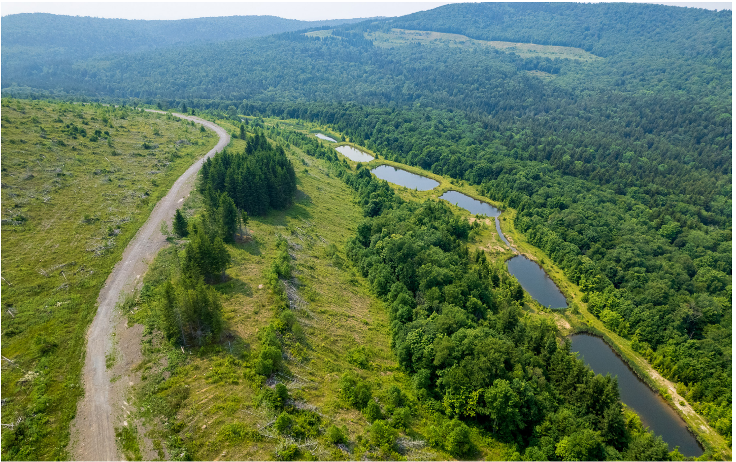
Aerial view of the ponds before work begins on their removal.
