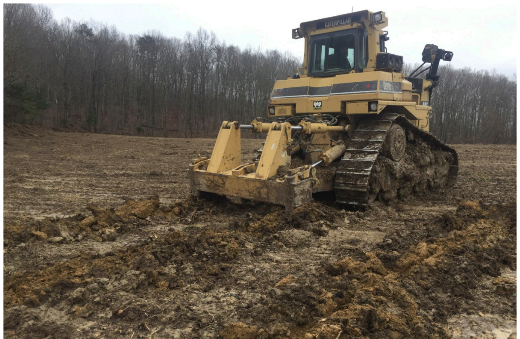
Heavy equipment is used to remove unwanted vegetation and decompact soil.
