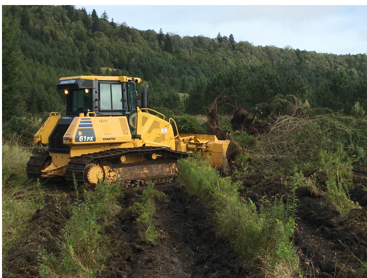
Figure 7. A Komatsu D61 bulldozer pushes felled trees across ripped ground.
