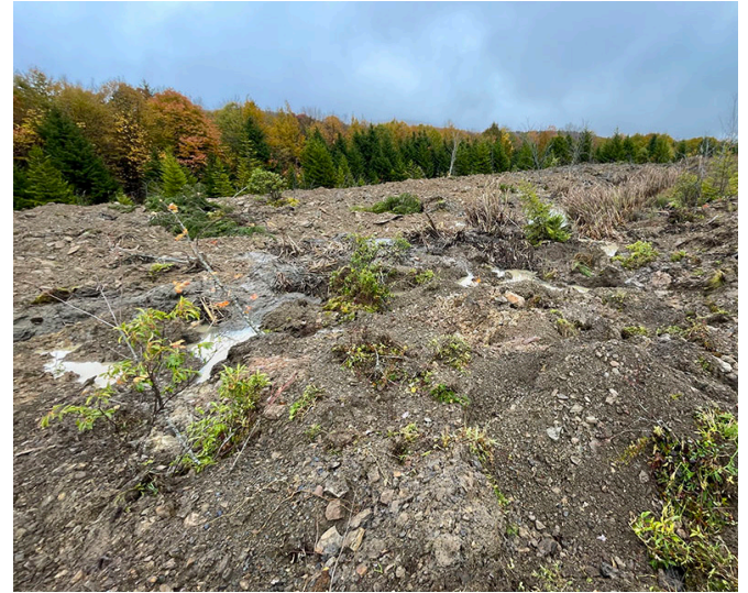
Left: Aerial view of the ponds before work begins on their removal. Right: Post removal landscape in an area where one of the ponds was decommissioned. Bottom: The downgradient berm of the pond is eliminated and pushed into the depression where water once stood.
