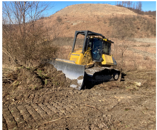
Fig. 4 — A small bulldozer removes autumn olive as well as the sod and seedbank prior to cross-ripping.
