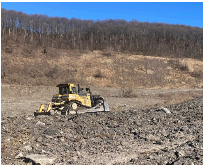
Fig. 5 — A bulldozer rips compacted soil in preparation for planting.
